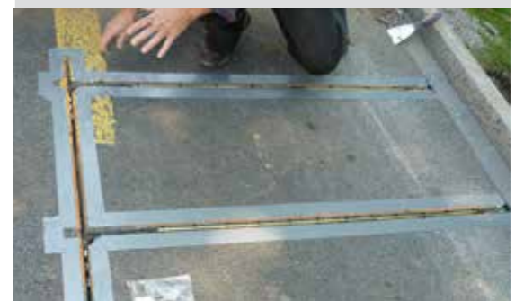
Installation of a fixed counting station with piezo technology. Only on smooth surfaces, no paving. Up to 5 m maximum width per lane.
